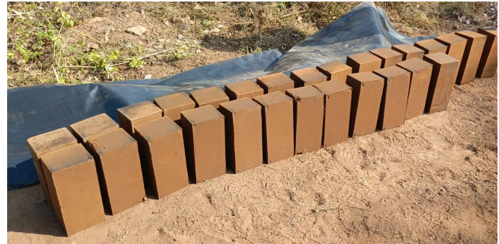
Production & Curing of SSB on the construction site
