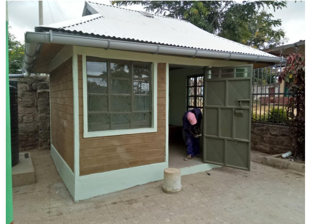
SSB house featuring rainwater harvesting
