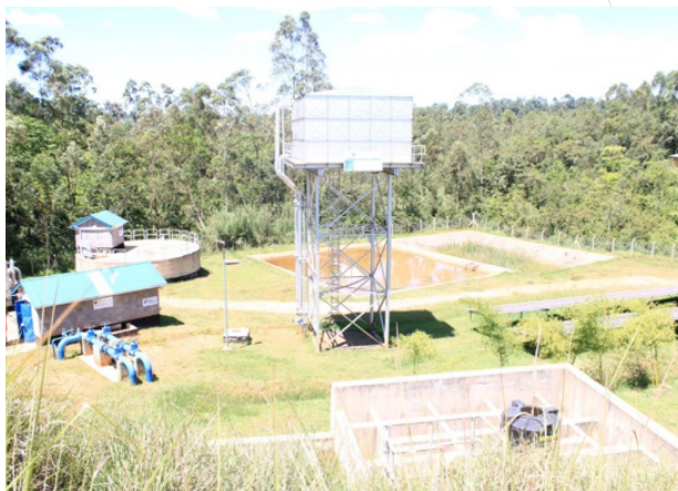
Figure 38: Lunyerere water project (Partly powered by Solar) energy)
