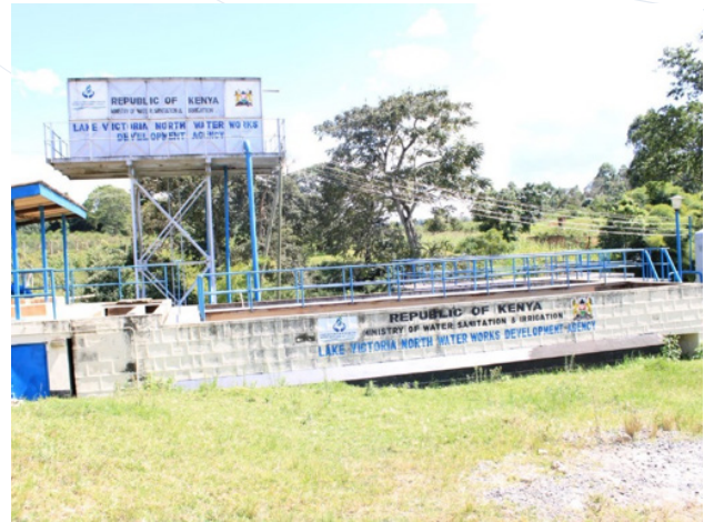
Figure 31: Kaimosi Hydropower Plant – water storage tanks (day 3)
