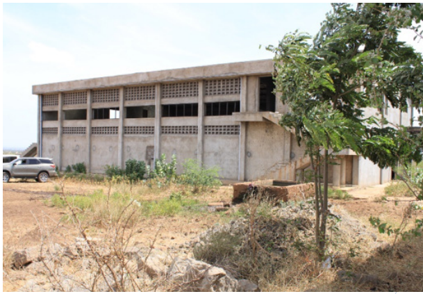
Figure 44: Uncompleted banana processing plant in Taveta
