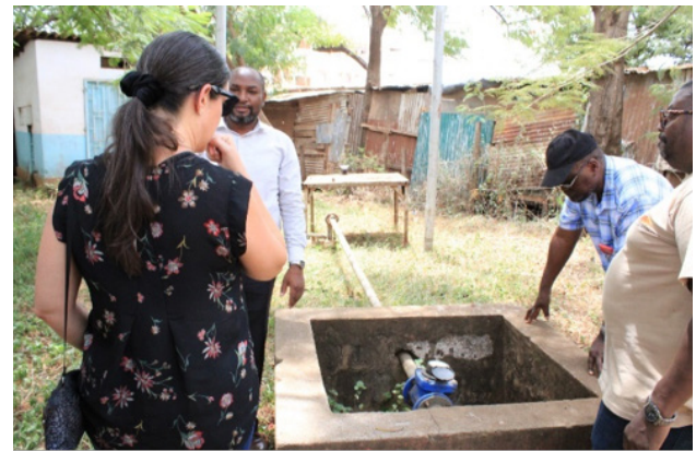
Figure 35: Borehole at Tavevo Water and Sewerage Company offices in Taveta (day 3)
