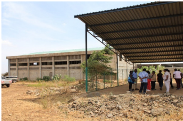
Figure 24: Site visit to the uncompleted banana processing facility at Taveta (day 3)
