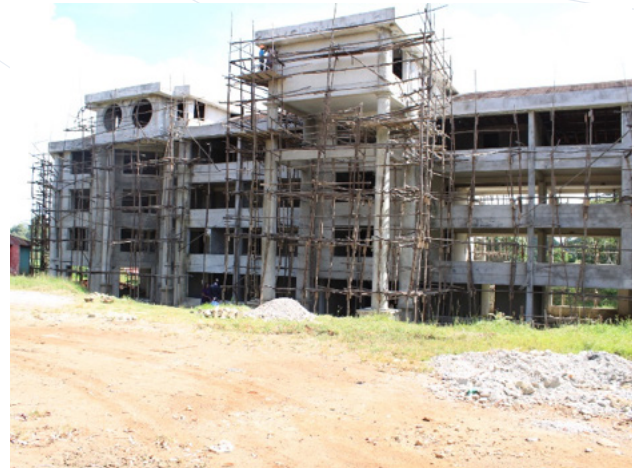
Figure 29: Site visit to New Governor's Office (day 3).
