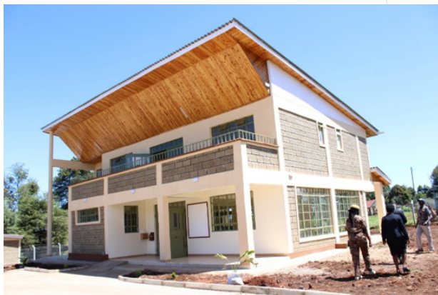
Figure 37: NEMA Green Point Building in Kapsabet Town
