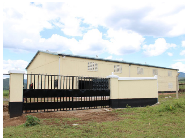
Figure 31: Site visit to Coffee Milling Factory Tinderet (day 2).
