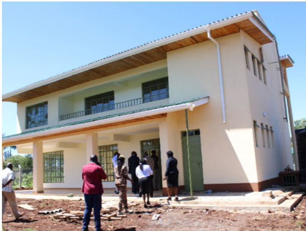
Figure 16: Site visit to NEMA green point building in Kapsabet - day 1.
