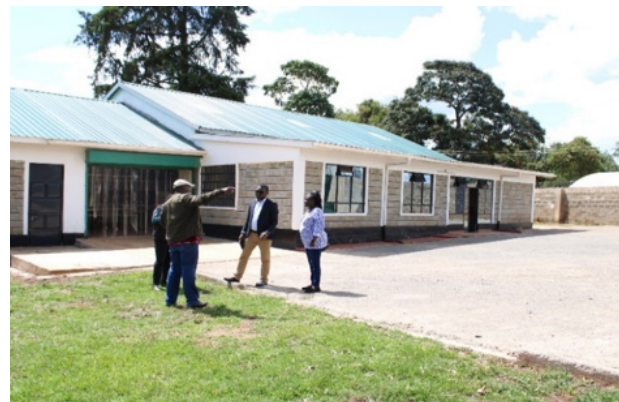
Figure 41: Nandi Poultry Slaughter House - exterior view
