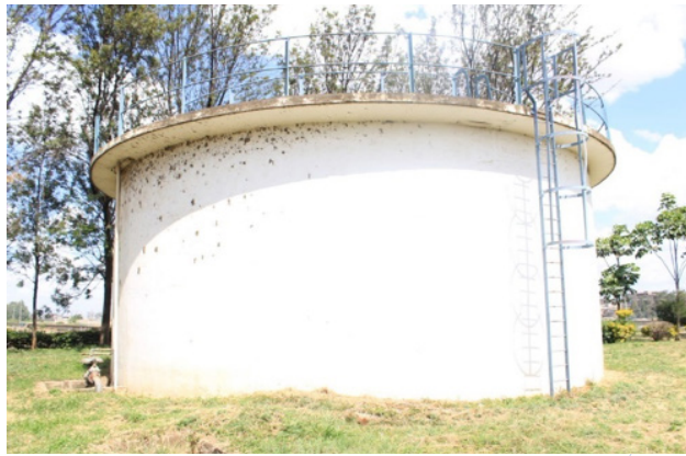
Figure 44: Kariobangi Sewerage Treatment Plant - Biogas storage tank
