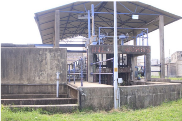
Figure 33: Site Visit to Kariobangi Sewerage Treatment Plant - Intake Facility (Day 3)
