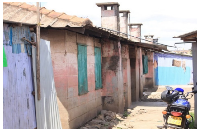
Figure 28: Site visit to County Government houses in Bahati Estate (day 3)
