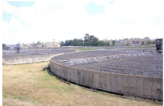
Figure 34: Site Visit to Kariobangi Sewerage Treatment Plant - Biological Sewage Water Pits (Day 3)
