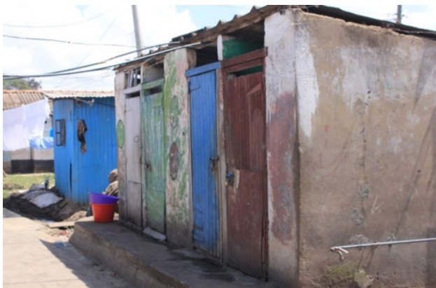
Figure 29: Site visit to County Government houses in Bahati Estate (day 3)
