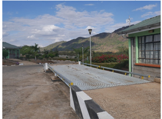
Figure 28: Makueni Fruit Processing Plant site visit (day 3)
