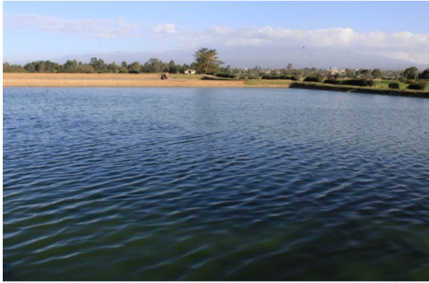
Figure 31: Nanyuki sewerage treatment plant (Day 4)
