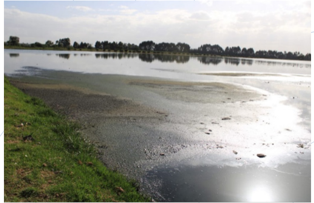
Figure 32: Drying sludge - Nanyuki sewerage treatment plant (Day 4)
