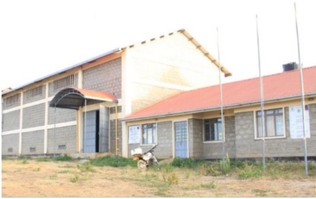
Figure 23: Laikipia Maize Storage Facility Kinamba (Day 3)
