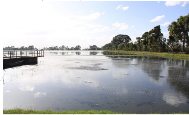
Figure 47: Nanyuki Sewerage Treatment Plant
