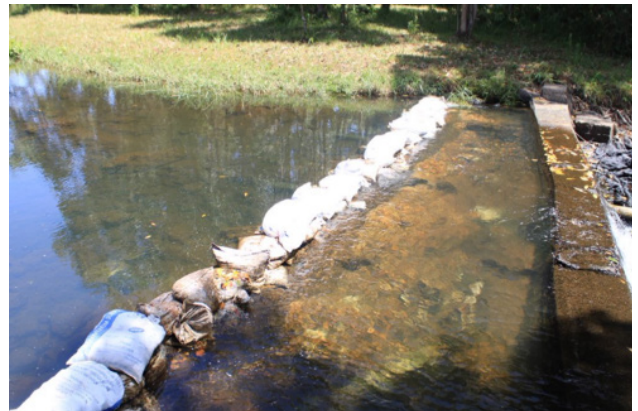
Figure 29: Thambana Dam proposed intake location - sandbags used to raise water levels (day 3)
