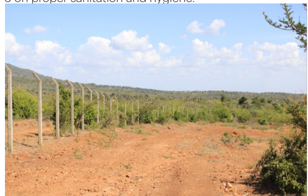
Figure 45: Kamwimbi Landfill – Perimeter fencing
