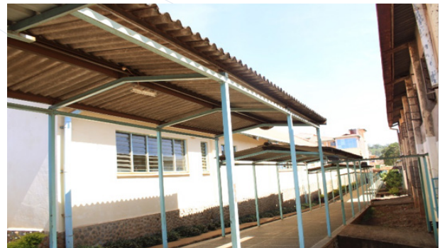
Figure 43: Embu Level 5 Hospital - Asbestos roofing at the general wing
