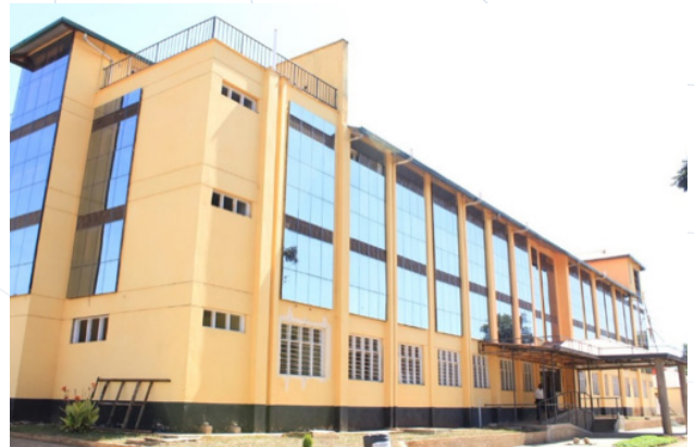
Figure 25: Embu Level 5 Hospital - private wing not operational (day 3)
