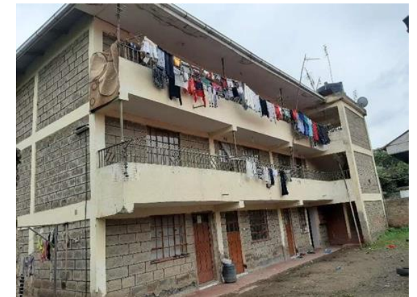
20 units financed by Large Sacco Ongata Rongai
